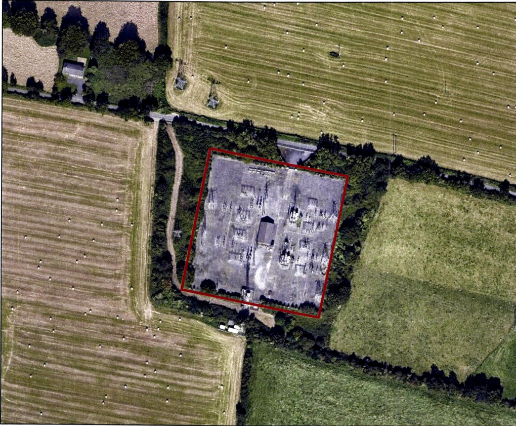
Figure 2-1 Fassaroe Substation Aerial Photo
